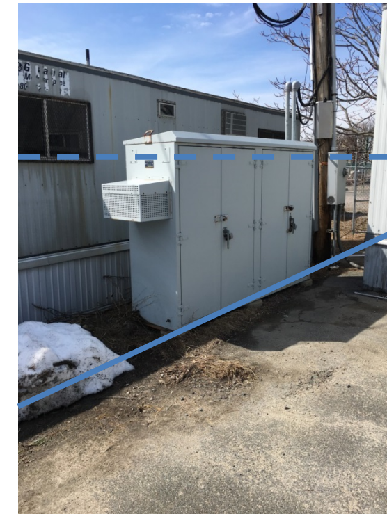
Figure 13: AC Power Feed Trailer Park
