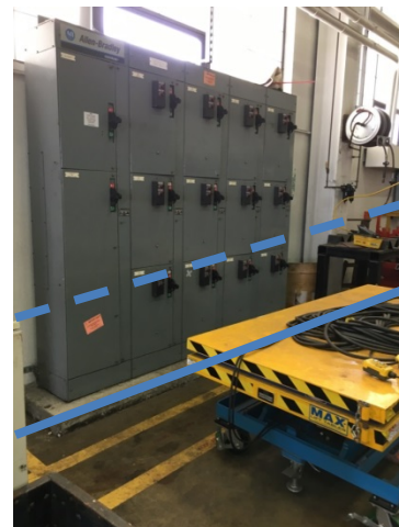
Figure 28: Maintenance Equipment – Barn Hoist Power/Controls
