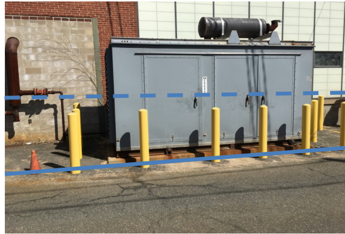
Figure 24: Building Systems – Emergency Generator
