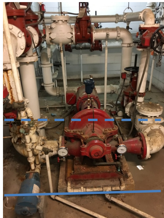
Figure 17: Building Systems – Barn Fire Pump
