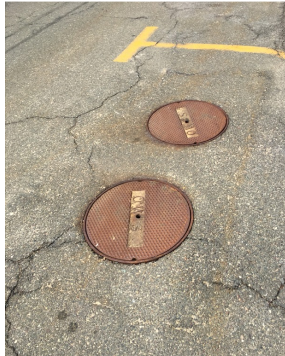
Figure 15: Oil Water Separator
