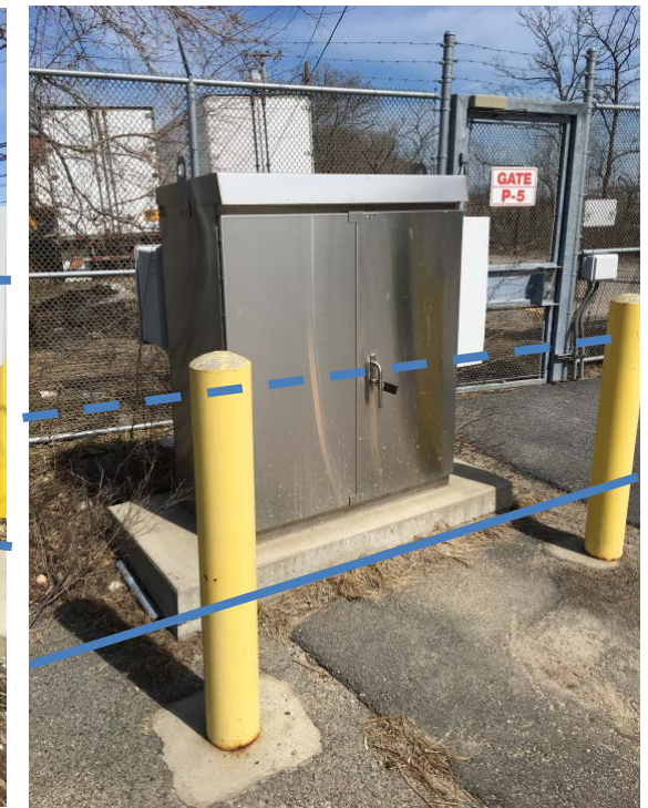
Figure 19: Blue Line Operations Yard Catenary Controller and Disconnect Switch
