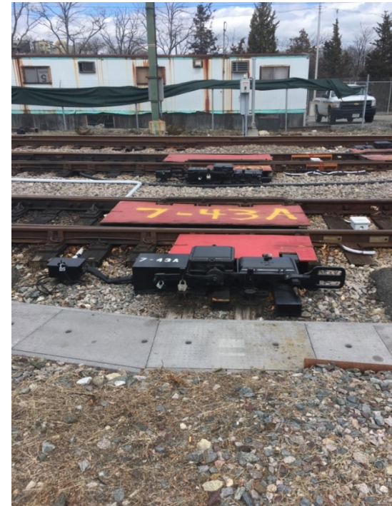
Figure 11: Blue Line Operations Signals and Power Switches entering the ROW
