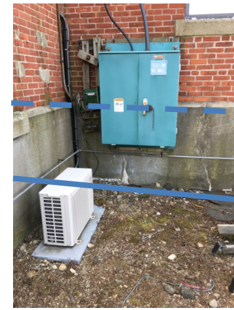
Figure 22: Maintenance Equipment – DC pull box
