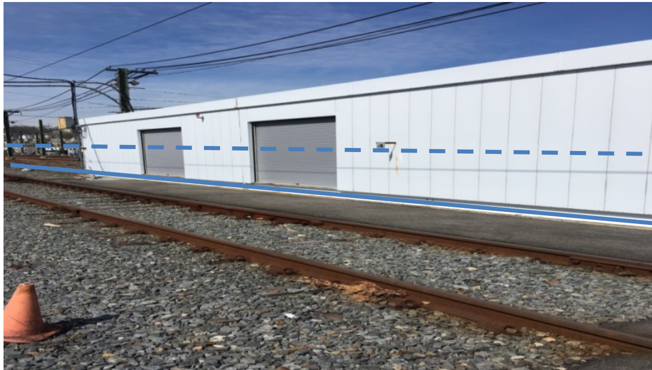
Figure 9: OH Car Yard Substation
