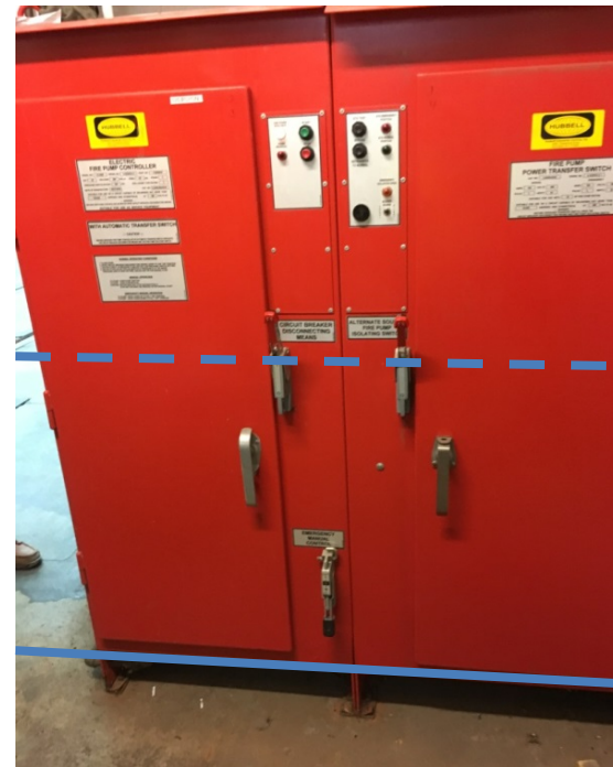
Figure 16: Building Systems – Fire Pump Control Unit
