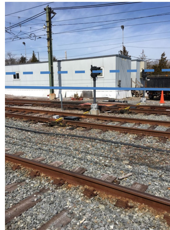
Figure 12: Maintenance Office Trailers
