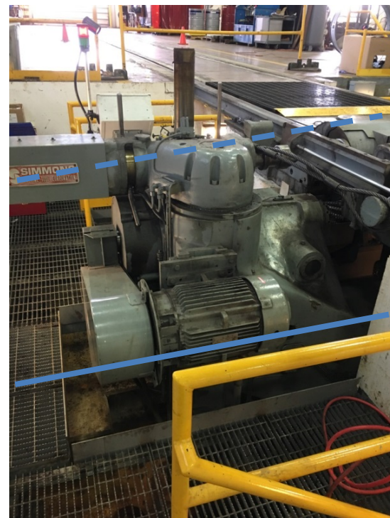
Figure 18: Maintenance Equipment – Wheel Truing Pit
