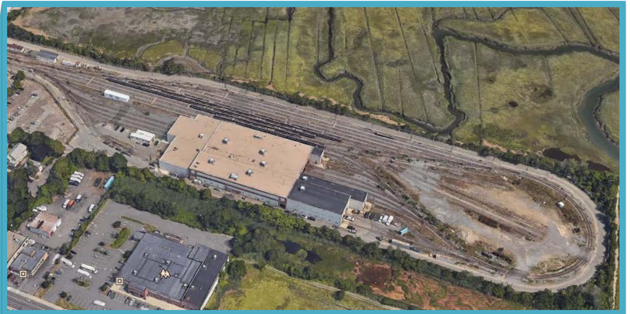
Figure 1: Orient Heights Car House and Maintenance Yard
