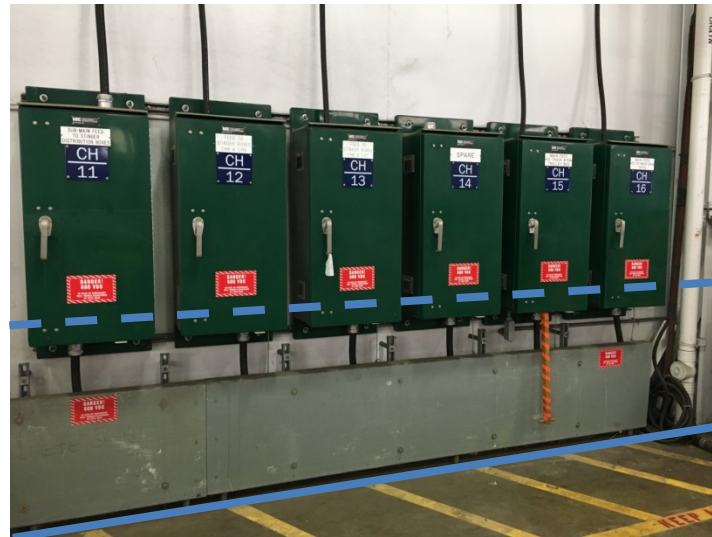
Figure 27: Maintenance Equipment – DC Power Disconnect
