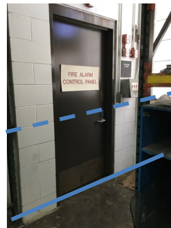
Figure 25: Building Systems – Barn Fire Control Panel Pump
