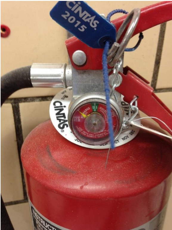
Quigley Memorial Hospital: Kitchen
