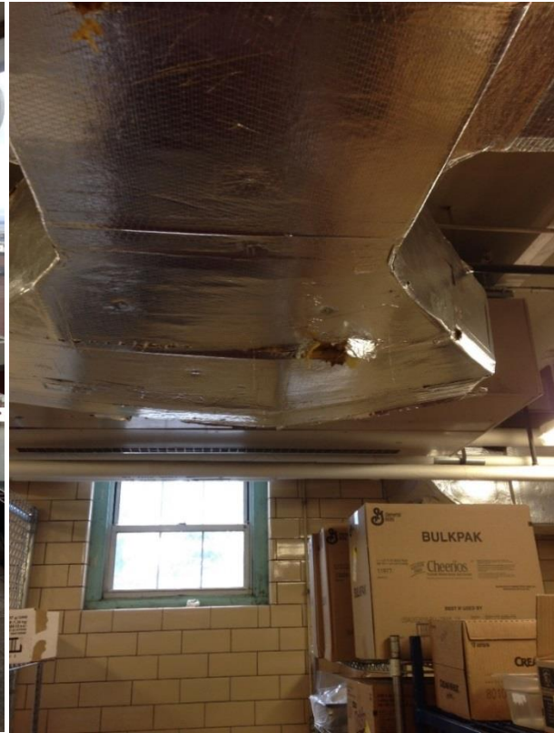
Quigley Memorial Hospital: Kitchen
