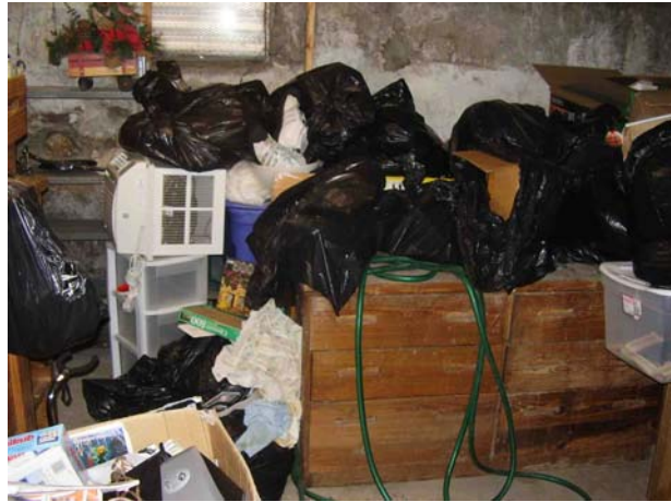
85 Alexander St. - Trash in basement
